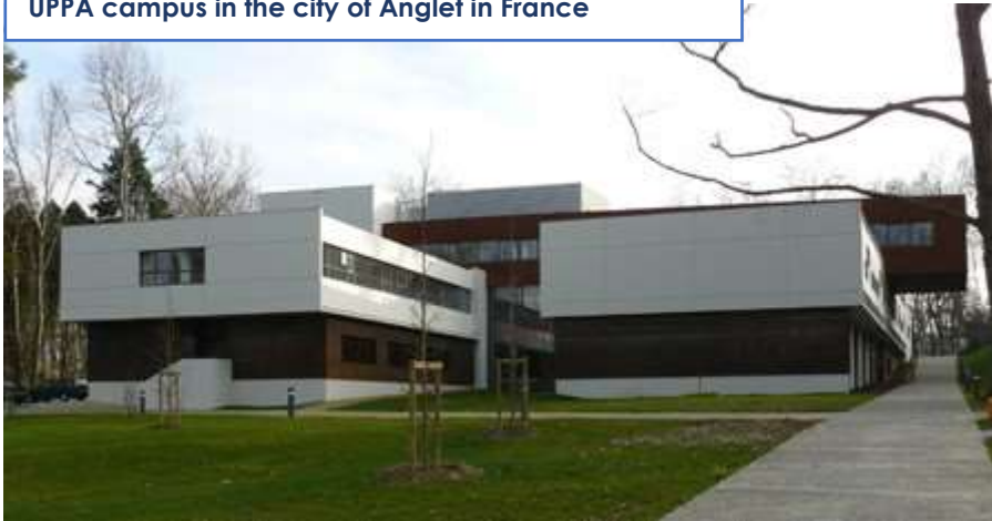
UPPA campus in the city of Anglet in France
